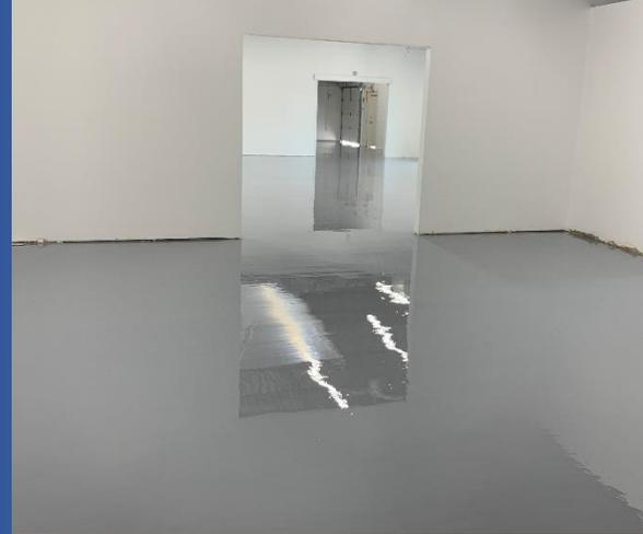
Often referred to as seamless floors or resinous flooring, epoxy floors are poured floors built for functionality and aesthetics. They are layered systems which are applied onsite with each layer having a specific purpose. The layers enable each resinous flooring system to be custom in design and to serve the demands of the exact area they are being applied.
